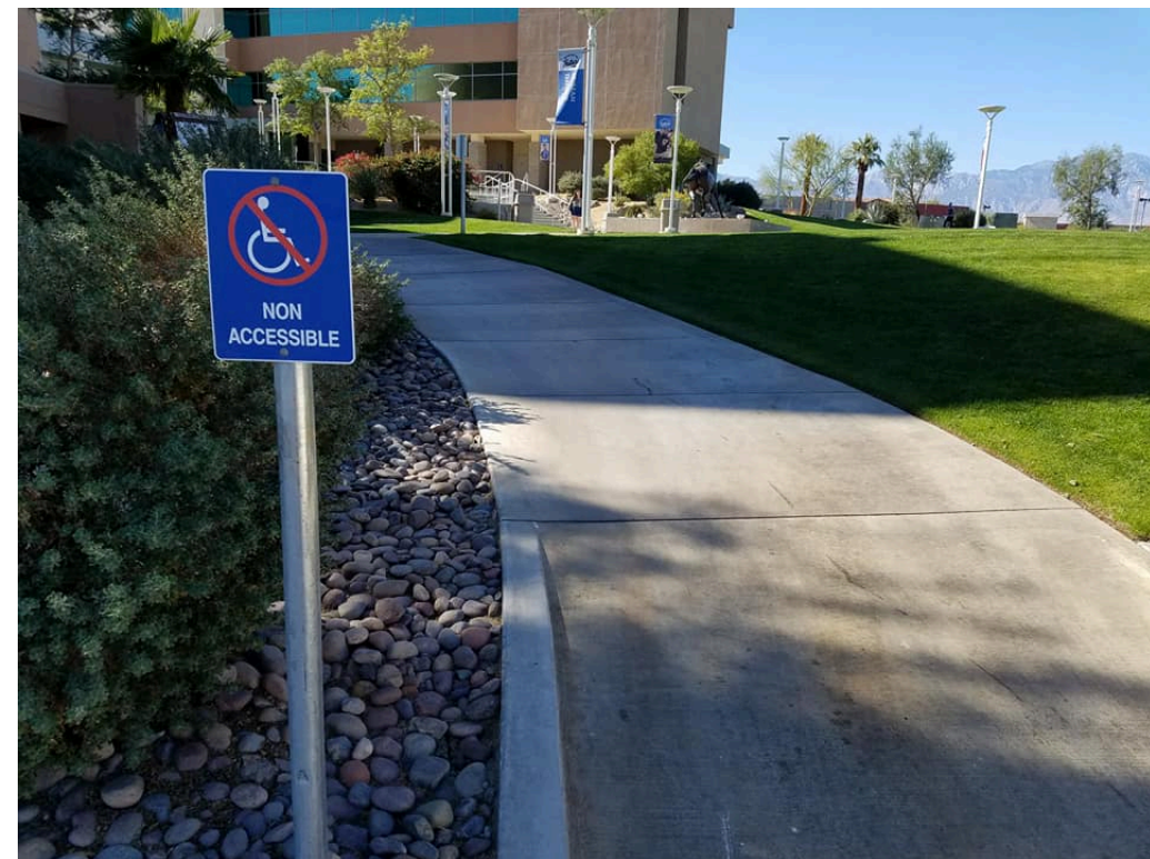
Picture 2: Ramp at Lot A entrance
