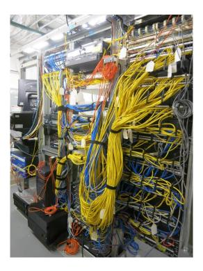
Each building is connected to the main server room with backbone copper and fiber cabling (multimode and single mode). Backbone cabling is routed in existing conduit duct bank pathways. See picture below of backbone conduit/cabling entering server room.
