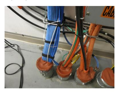
Most of the telecom rooms are also used for spare equipment and cabling storage. The telecom rooms would gain proper clearances and future expansion space if the non-active equipment, spare equipment and cabling was removed.
