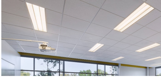
acoustical ceiling with controllable LED lighting
