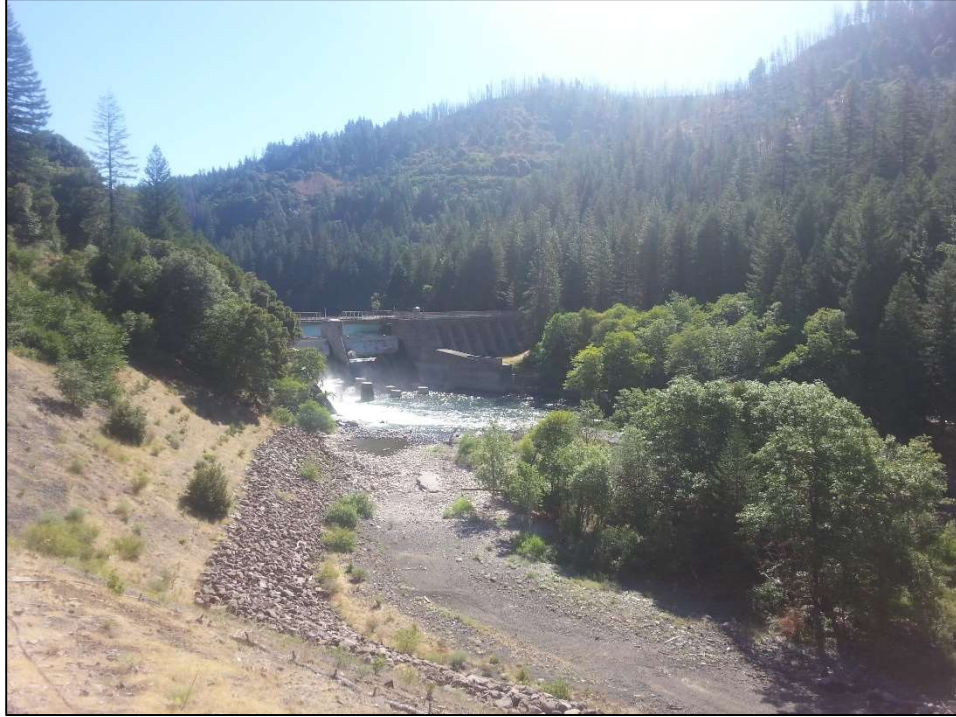
Figure 2. Pit River hydroelectric dam called the Pit 2.
