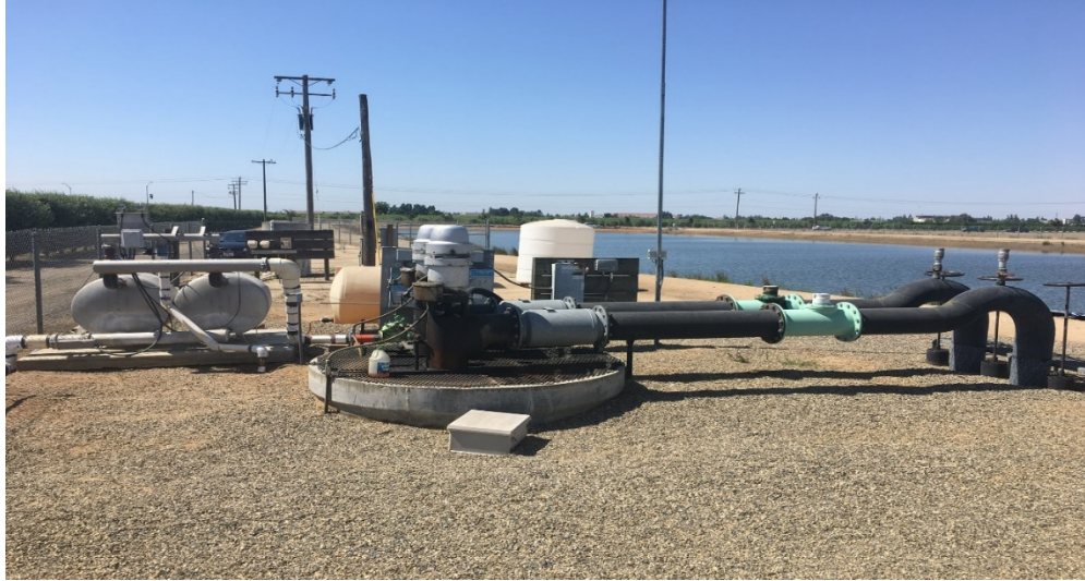
Figure 4: Irrigation Pump at Olive Field
