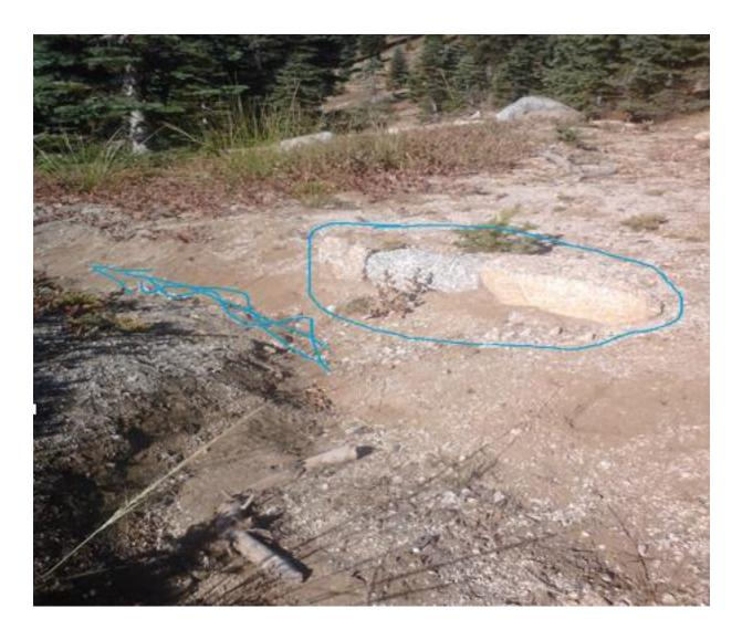
Picture 1: Water Bar on decommissioned trail causing large runnel
