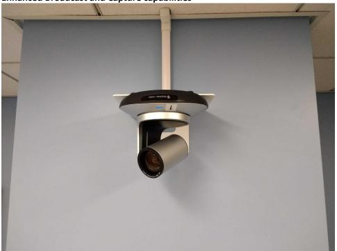
Three separate HD cameras with full Pan-Tilt-Zoom support have been installed so remote audiences need not feel 'stuck' in the corner. They are positioned in the room at key vantage points to maximize presenter as well as audience views.
