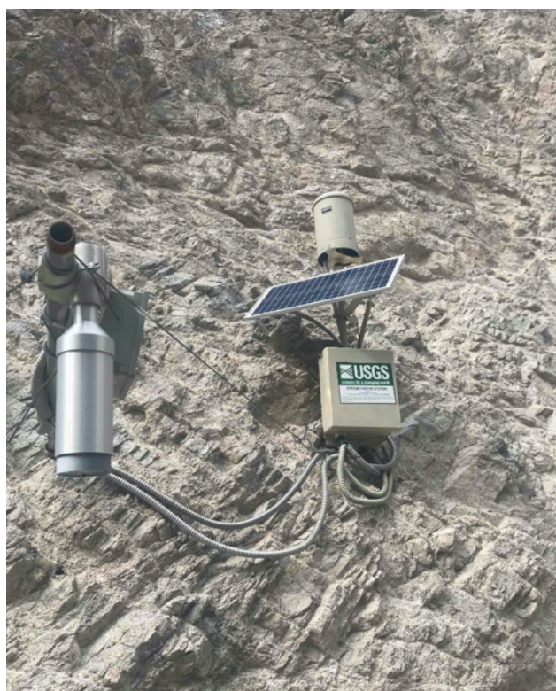
Figure 5. Rain gauge (top), solar panel, control box, and laser scanner (left) at Chalk Cliffs. Laser used to determine stage (depth) of flow and, hence, sediment volume that passes station per time increment.
