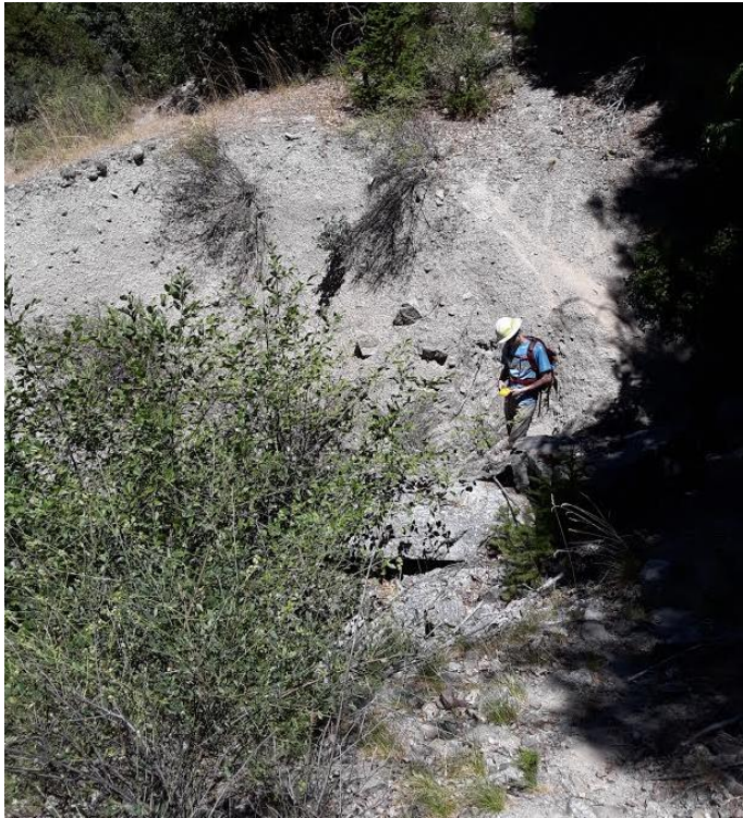
Figure 4. One of the hydrology intern is used as scale to capture the overall size of the culvert washout on the road. The intern is at the very bottom [center]of the washout. 2018
