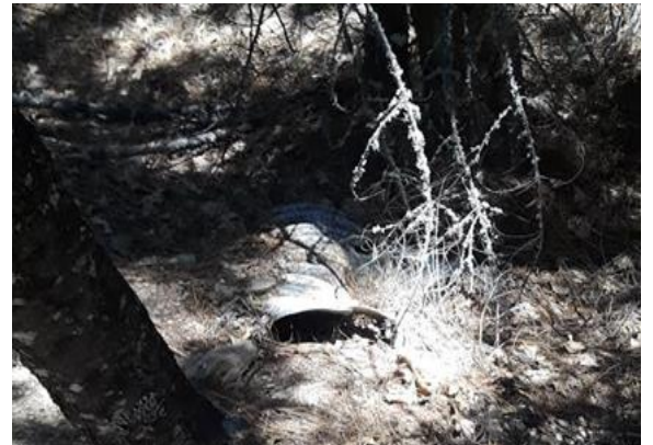
Figure 5. A buried culvert can potentially compromise a fully functional stream or cause road erosion during heavy rainfall. 2018
