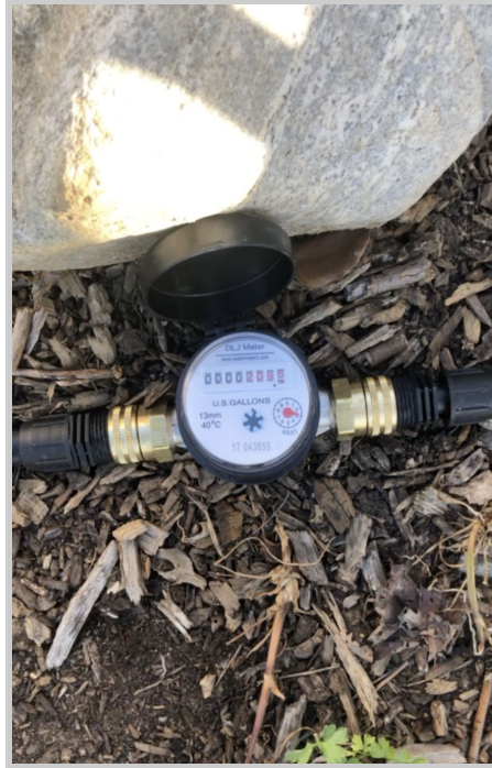
Figure 3. Installed water meters
