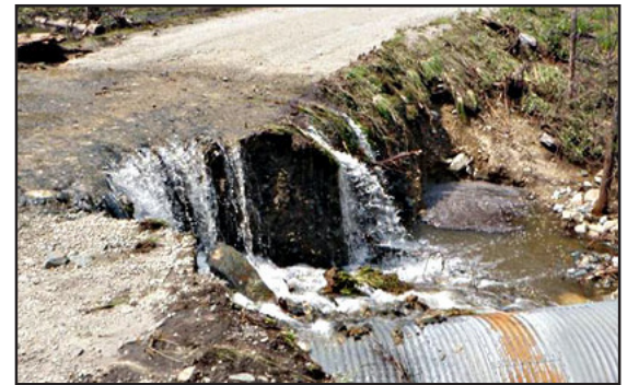
Fillslope erosion at the outlet due to sheet flow over the road surface
