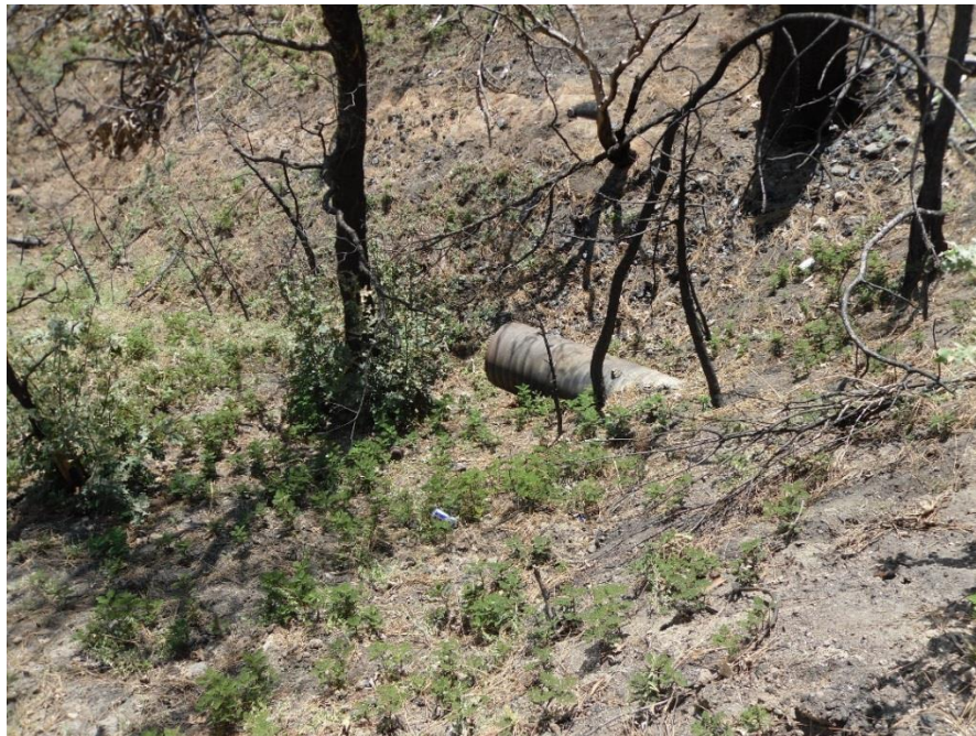
Figure 3: Culvert outlet with a shot gun. Protocol for culverts included measuring the culvert length, diameter, and outlet drop.
