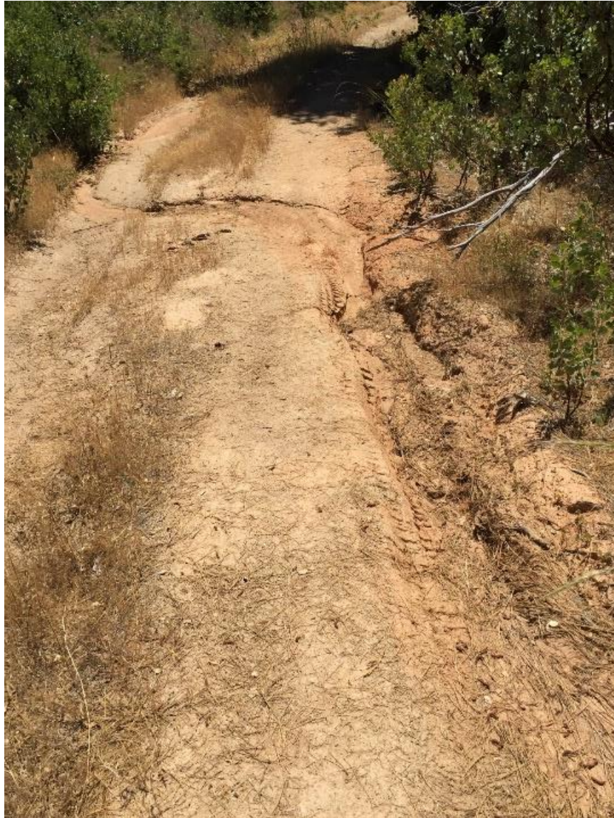
Figure 4: Road 10S090 is a good example of a hydrologically connected road segment with a failed waterbar and rills developing on the right side of the photograph.
