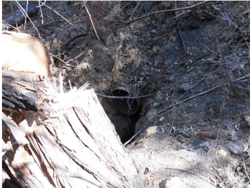
Figure 2: Culvert outlet, sometimes hidden or buried under fallen trees, debris or vegetation.
