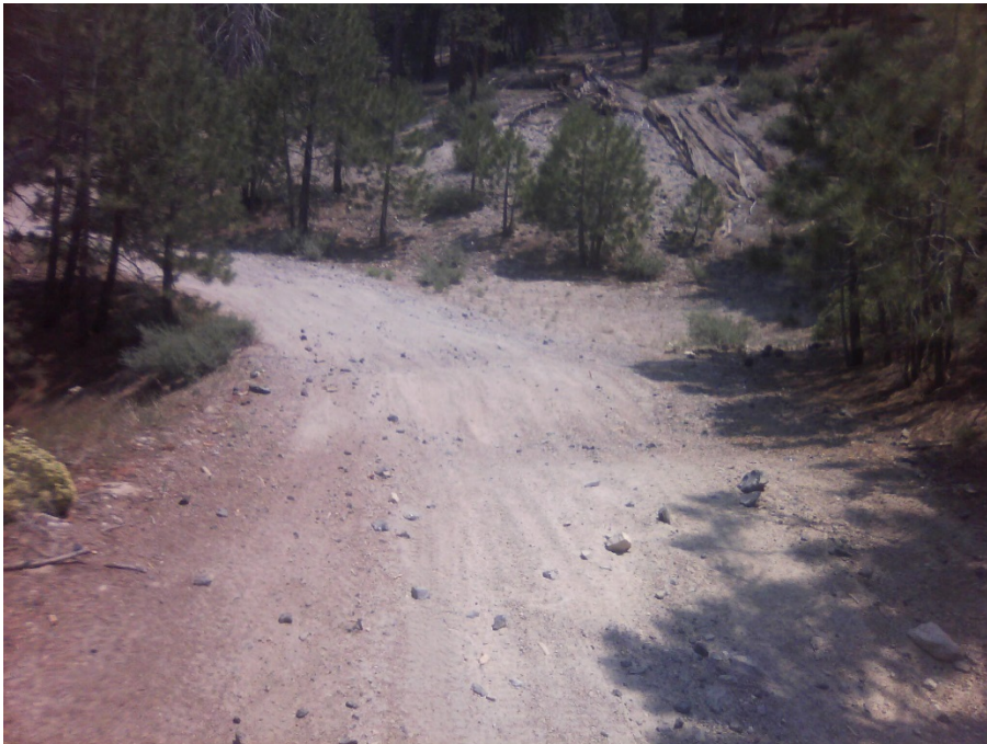
Figure 2. Another road that was showing little signs of erosion.
