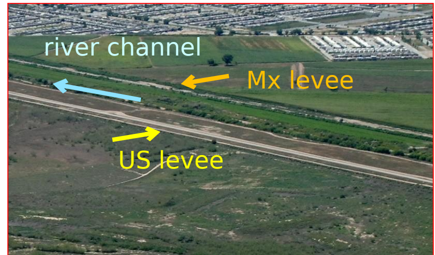
Rectified channel and levees
