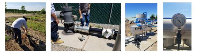
An important part of an irrigation system is the filtration station. The filter station is where water gets filtered before being pumped to the field and includes the chemigation system. NRCS requires that a filter station include pressure release valves in case of emergency, a pressure gauge both upstream and
