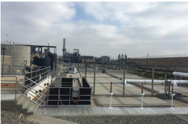
Figure 5. Water Treatment Facility
