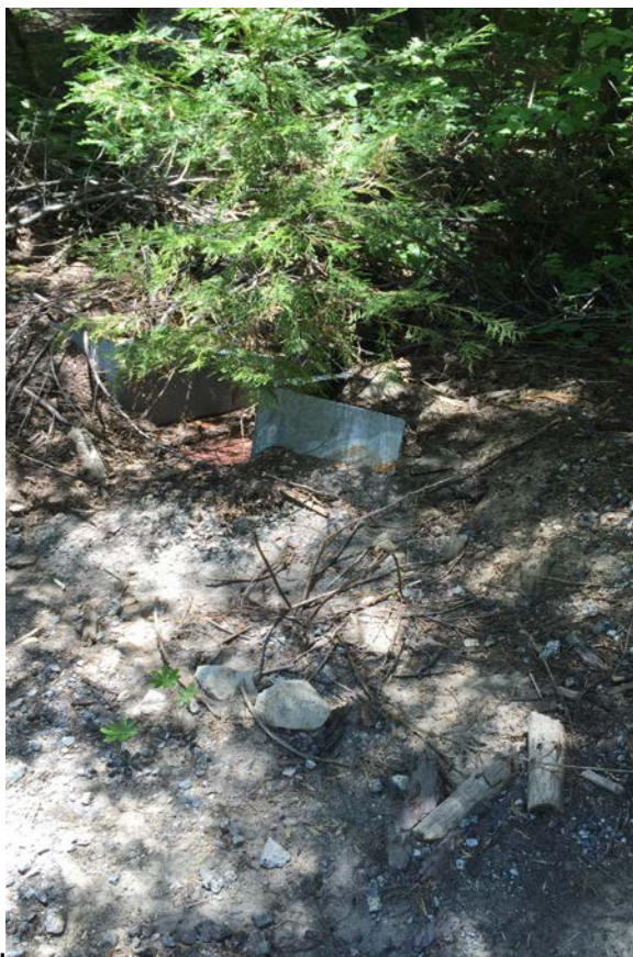
Figure 4: Overside Drain filled with debris.
