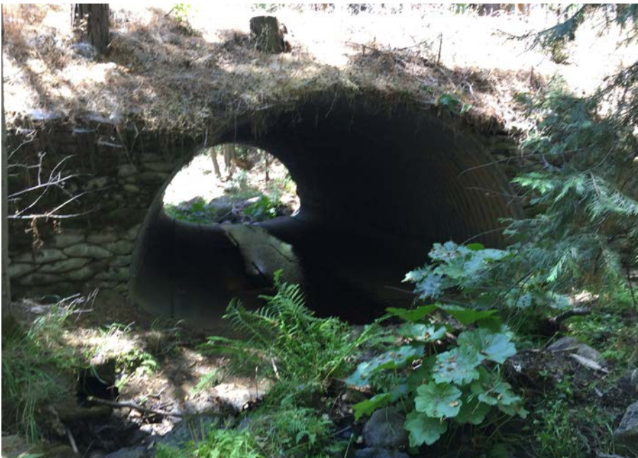
Figure 2: 100inch culvert near Bretts Mill WorkStation.
