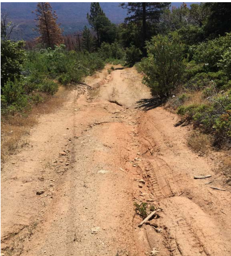
Figure 3: Segment of Road 10S090, showing signs of surface erosion
