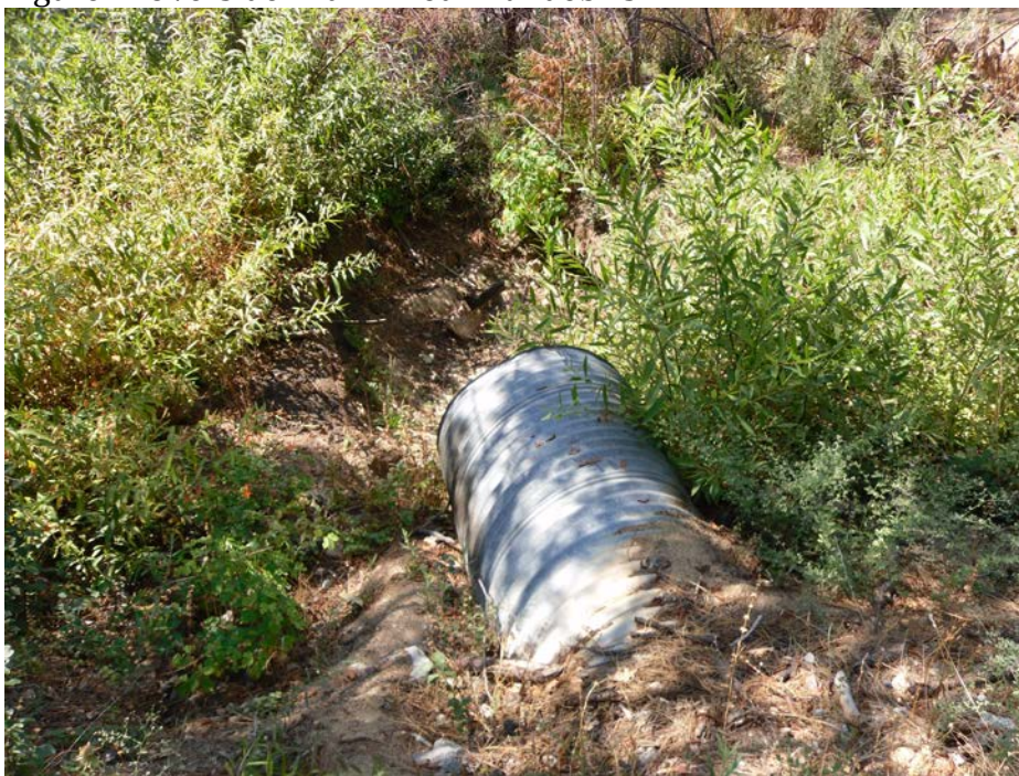
Figure 5: Shotgunned culvert off roadside with and outlet drop.
