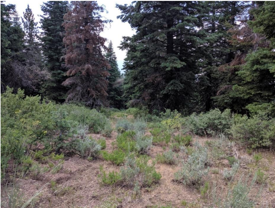
Picture that shows a level 2 maintenance road needing medium vegetation clearing and surface blading.
