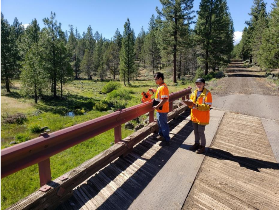
Picture showing engineering interns assisting bridge inspector with measuring potential scouring and writing report. On the left is intern David Phanthavady, and on the right is Alicia Nam.
