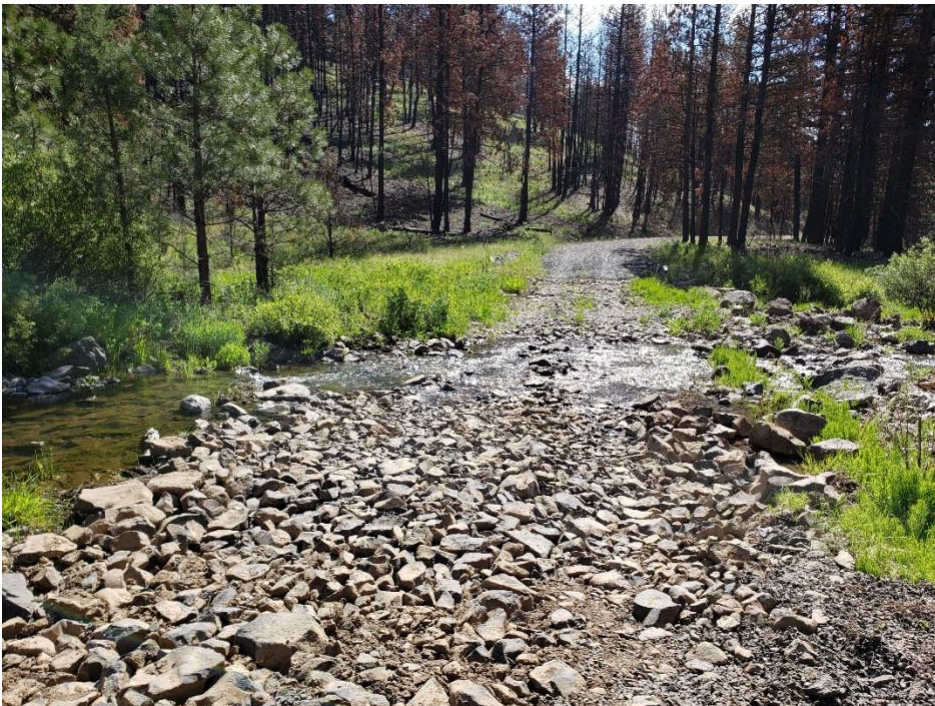
Picture that shows a stream crossing that needs a culvert or vented Ford installation to protect potential fish-bearing stream.
