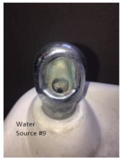
Water Source #7: Moldy, dusty, rusty Water Source #8: Moldy, dusty, rusty Water Source #9: Moldy, rusty, dusty, lime
