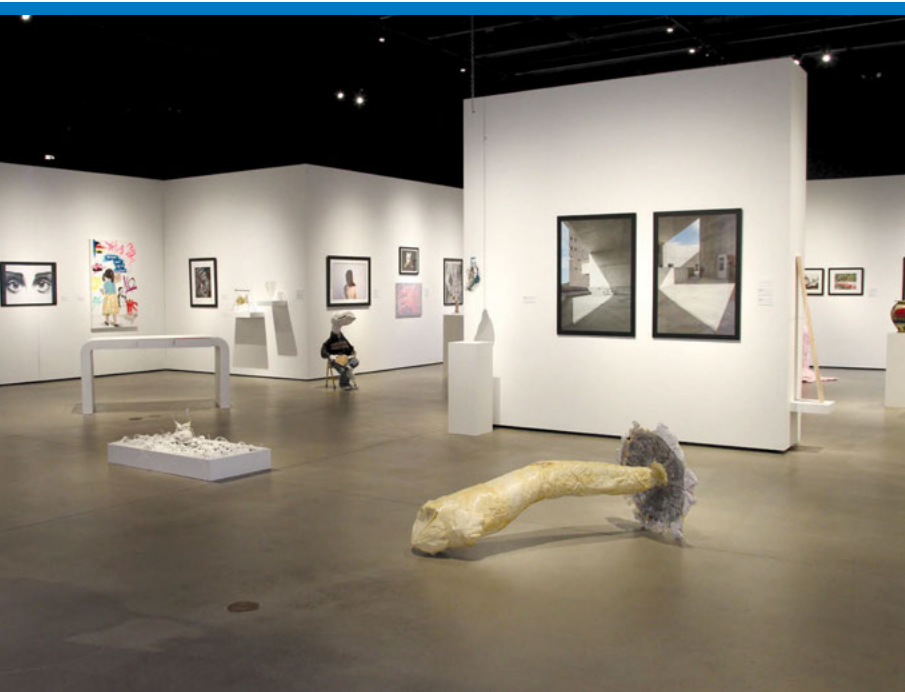
New LED lighting reduced wattage use in this museum space from 75 watts down to 13, and they run much cooler than the halogen lights they replaced.
