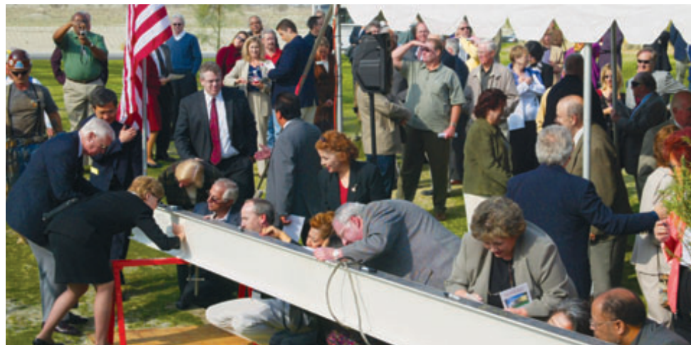
HALFWAY POINT — Guests signed the final beam in indelible ink before it was hoisted in place atop the two-story Indian Wells Center. Construction will be completed in time for the beginning of the academic year this fall, when PDC will consolidate all of its classes and programs at the new campus. Some classes remain in temporary buildings at College of the Desert.
