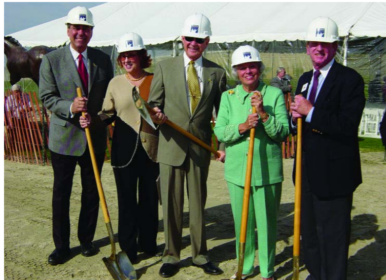
LET THE BUILDING BEGIN — Among the 200 guests at the groundbreaking for the desert campus's second building were (from left to right) CSUSB President Albert Karnig, Carol Adney, PDC director of development, Dick Oliphant and Betty Barker, co-chairs of the PDC campaign committee, and Peter Wilson, PDC dean.
