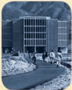
Library collection moved to new five-story library-classroom building
