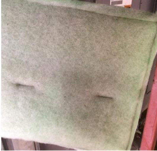
MZ 3 poly tacky filter with trace dirt loading
