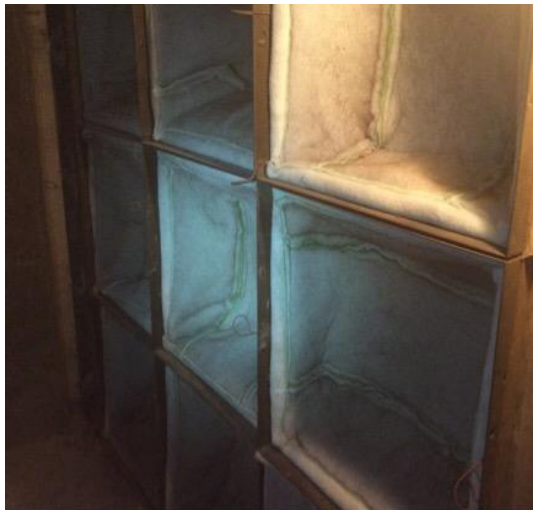
AHU 6 polytacky filters with trace dirt loading
