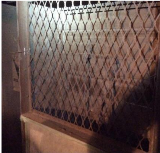
AHU 5 - O/A dampers closed
