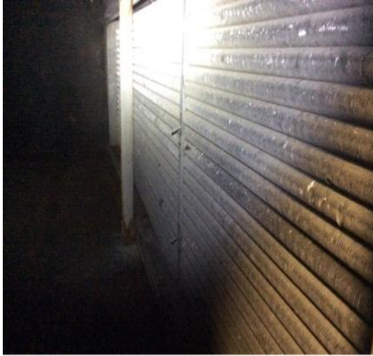
MZ 1 - coils with trace dirt loading and rust.
