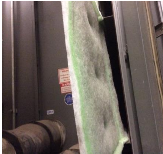
Wedge AHU 2 - polytacky filter with trace dirt loading
