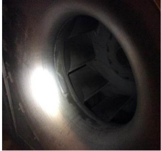
Wedge AHU 1 - A/S fan with trace dirt loading and rust on the inlet & housing.
