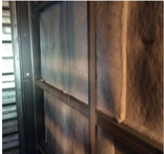
Wedge AHU 1 - polytack filters with trace dirt loading.
