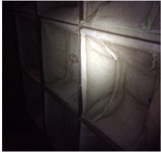
MZ 1 - Poly tacky filter with trace dirt loading
