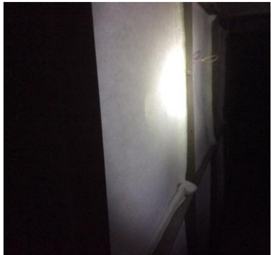
MZ 4 - poly tacky filters with trace dirt loading
