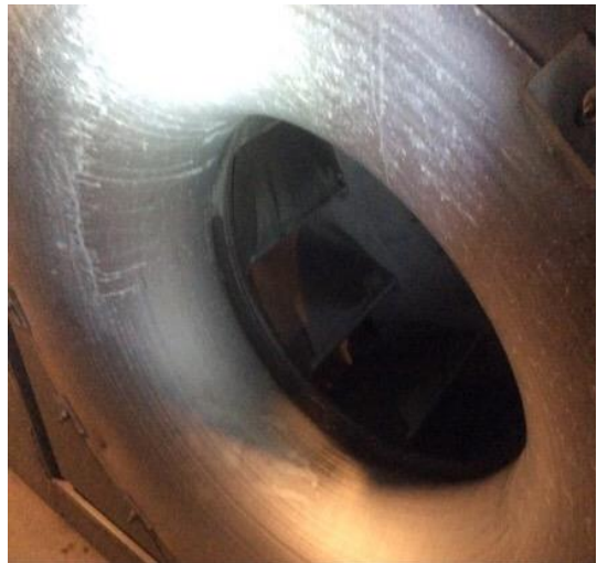
Wedge AHU 3 - A/S fan with trace dirt loading and rust on the inlet & housing
