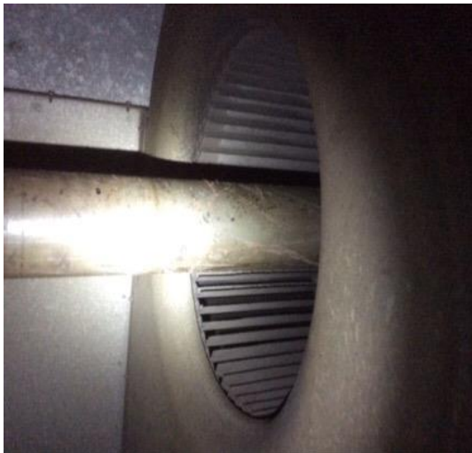
MZ 1 - A/S fan with trace dirt loading and rust on the inlet and housing.
