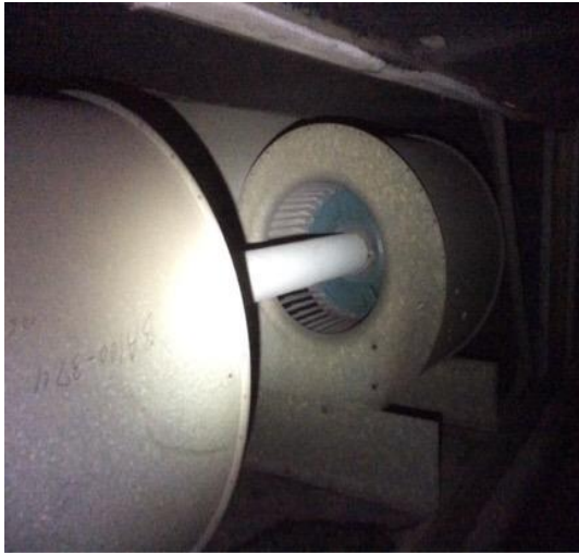
MZ 4 - A/S fans with trace dirt loading & rust on the inlet & housing
