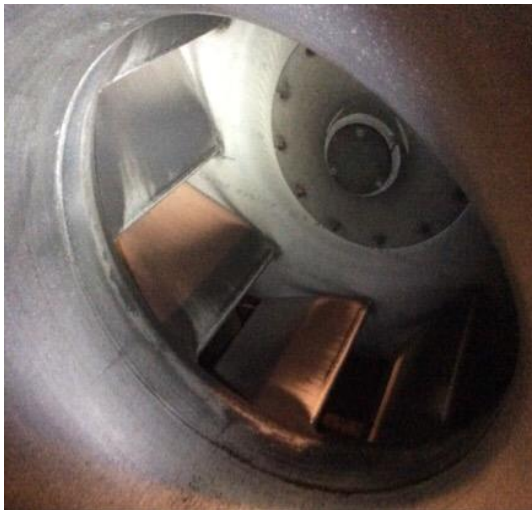
Wedge AHU 2 - A/S fan with trace dirt loading and rust on the inlet.
