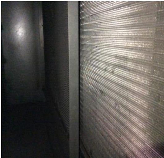
MZ 3 - coils with trace dirt loading
