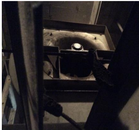
AHU 5 - A/S fan light dirt loading and trace rust on the inlet and housing
