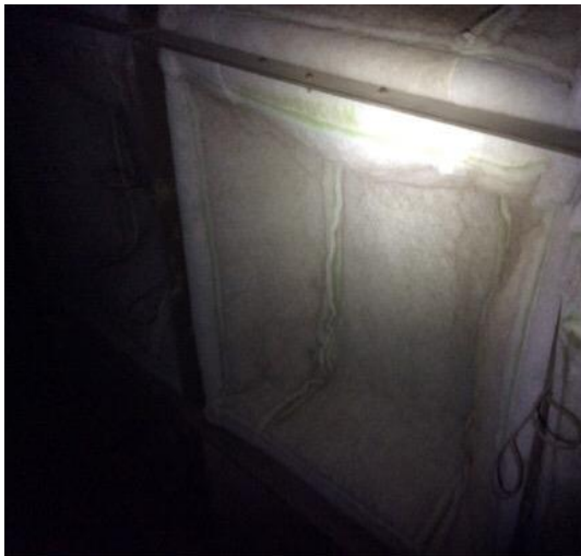
MZ 2 - poly tacky filter with trace dirt loading
