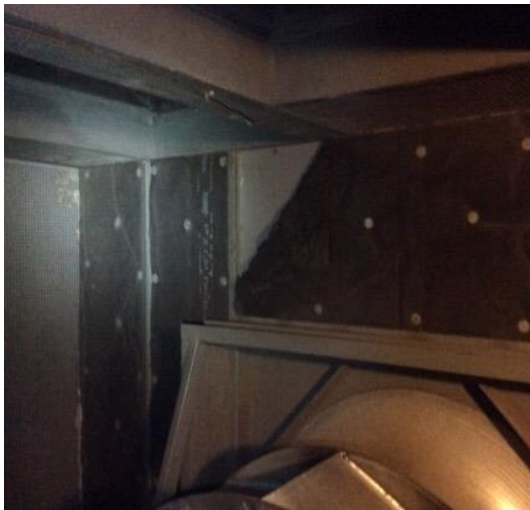
Wedge AHU 3 - torn insulation in fan chamber
