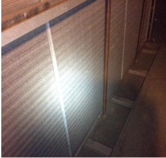
Wedge AHU 1 - coils with trace dirt loading and rust.
