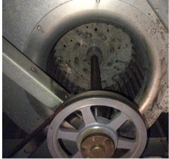
MZ 3 - A/S fan with trace dirt loading on the inlet & housing.
