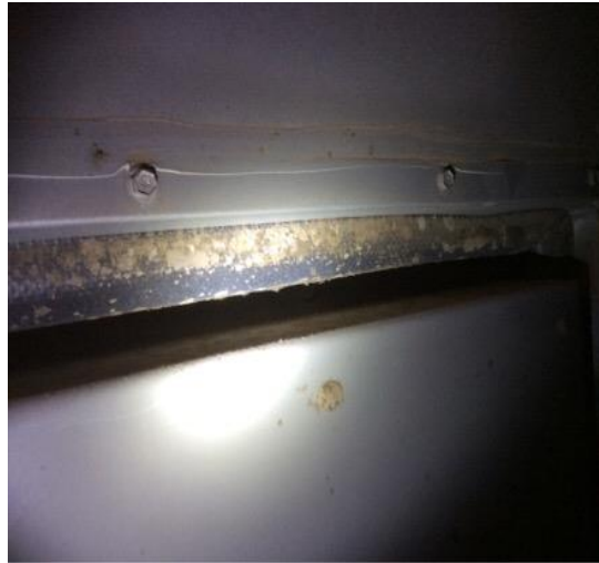
Wedge AHU 2 - suspect microbial growth on the vibration collar on the A/S fan
