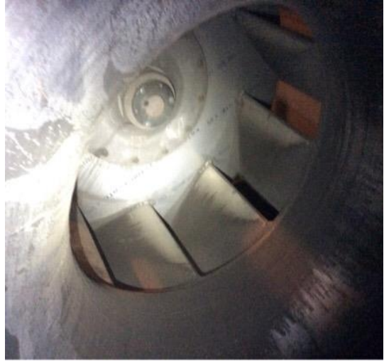
Wedge AHU 2 - R/A fan with trace dirt loading and rust.
