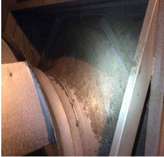
Wedge AHU 2 - suspect microbial growth on the back side on the A/S fan
