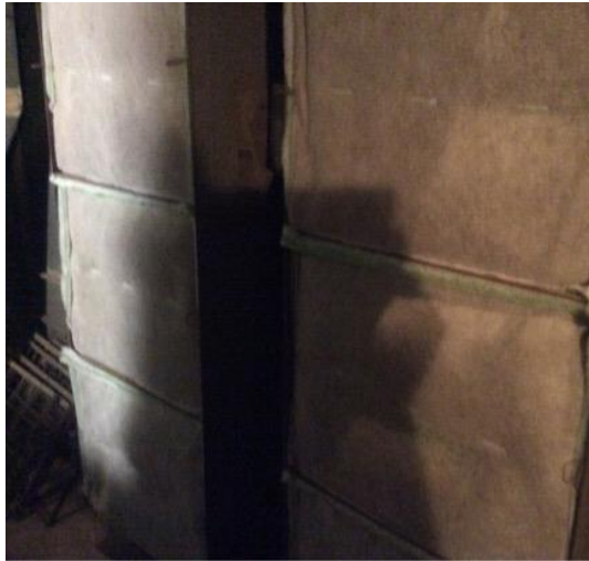
AHUs 5 & 6 - polytacky filters with trace dirt loading on O/A dampers
