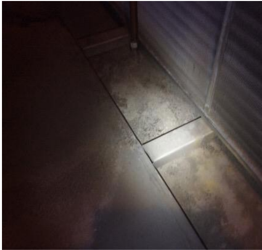
Wedge AHU 2 - condensate tray with trace dirt loading and rust.
