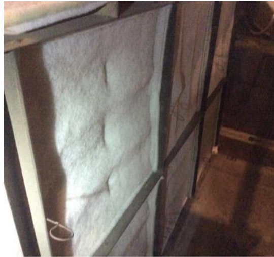
AHU 5 - polytacky filters with trace dirt loading
