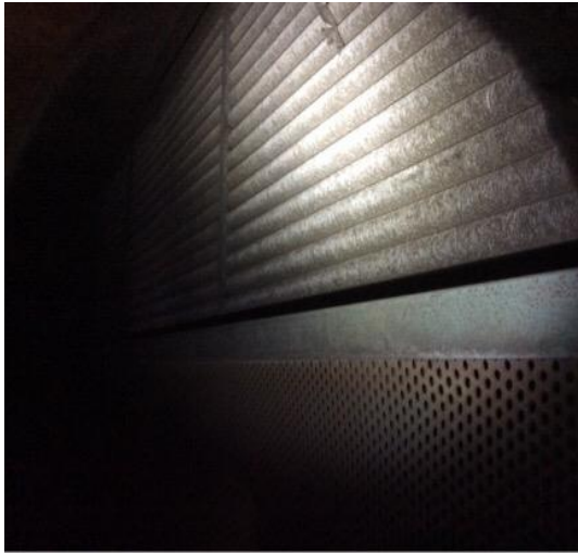
MZ 2 - heat coils with trace dirt loading & rust
