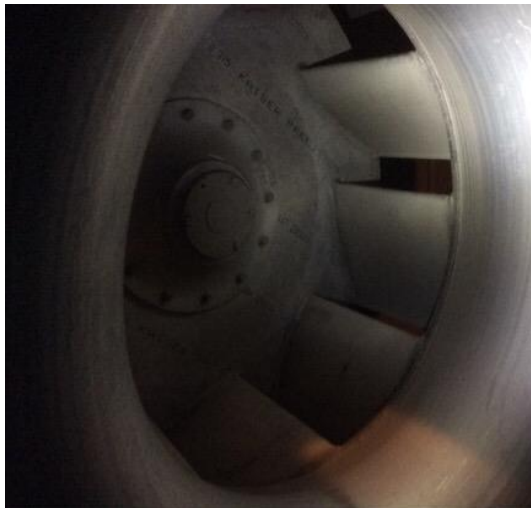
Wedge AHU 3 - R/A fan with trace dirt loading and rust on the inlet and housing.
