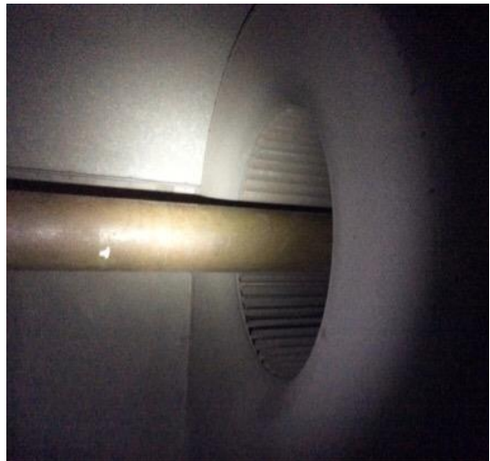
MZ 2 - A/S fan with trace dirt loading & rust on inlet & housing
