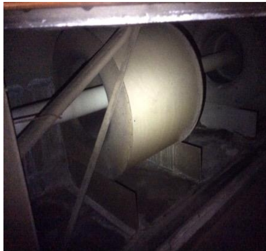
AHU 5 A/S fan with light dirt loading and trace rust
