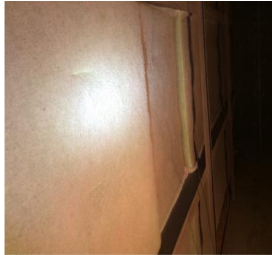
Wedge AHU 3 - polytacky filters with trace dirt loading.
