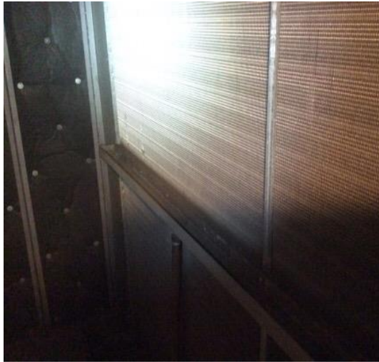
Wedge AHU 3 - cooling coils with trace dirt and rust loading.
