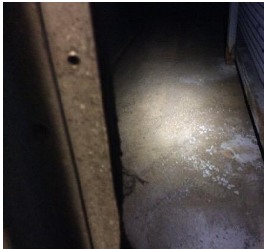
MZ 1 - condensate tray with moderate dirt loading and trace rust.
