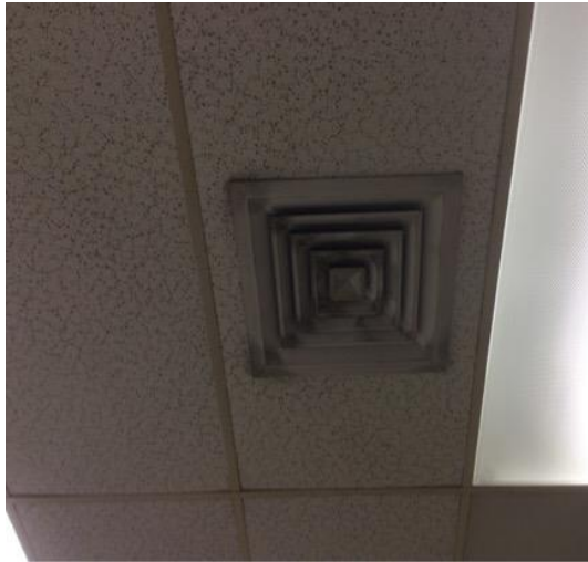
2F Classroom 214 air diffuser with trace/light dirt loading.
