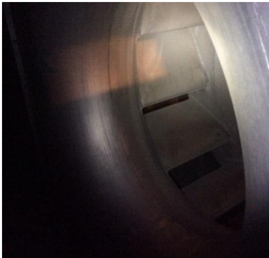
Wedge AHU 1 - R/A fan with trace dirt loading and rust on the inlet and housing
