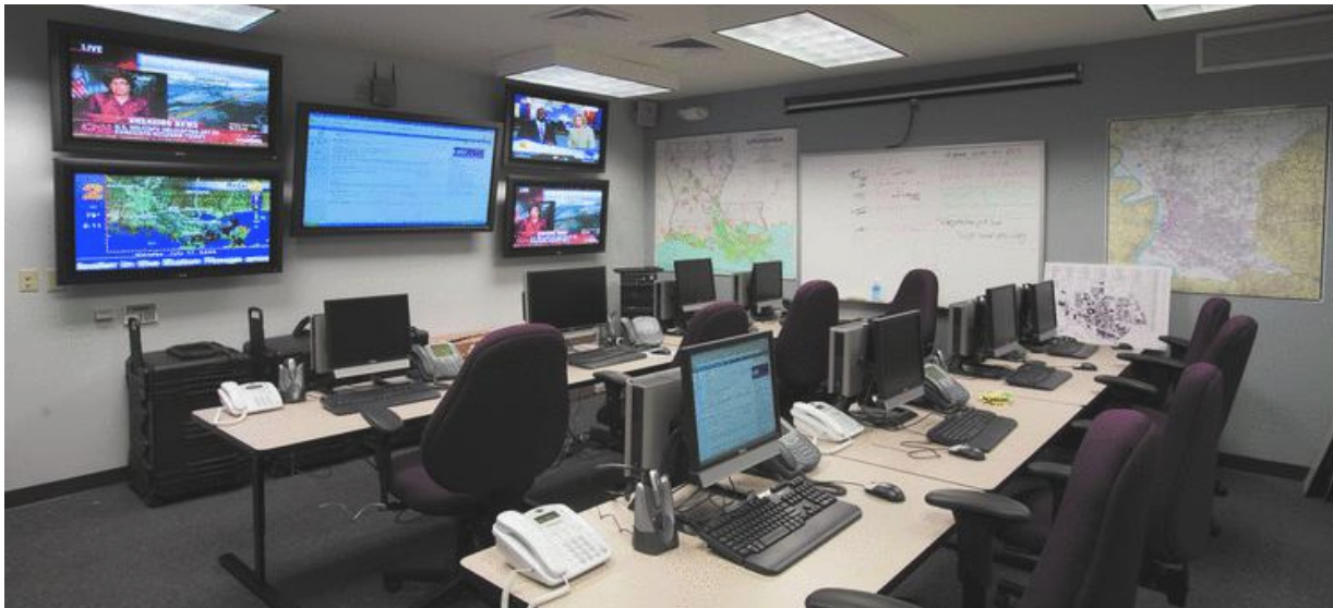
University Emergency Operations Center - A long term security infrastructure objective for the CSUSB campus.
