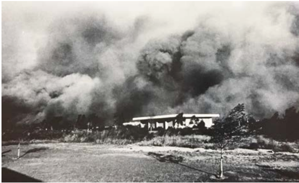
Fire resiliency has, and continues to be, a key concern at CSUSB. Above, the 1980 Panorama Fire damaged campus buildings.
