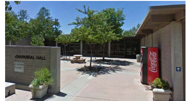
Chaparral Hall, Sierra Hall, and the current Administration building are among the oldest structures on campus and are the only buildings in this plan proposed for long-term replacement.
