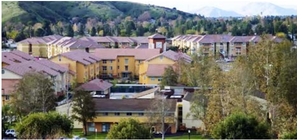
Existing residential buildings on campus are primarily 2 to 3 levels
