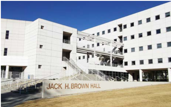
Campus building with poor accessibility
