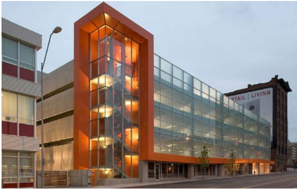
The tower of for each parking structure emphasizes entries to stairways and elevators. Solar roof panels are also provided on the top parking deck.
