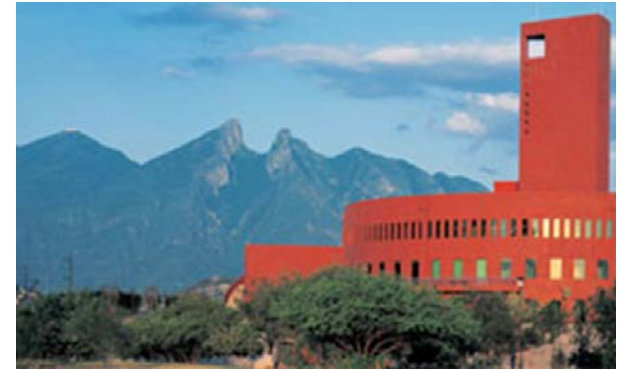
Recommended Example: Use of warm saturated colors for building exteriors
