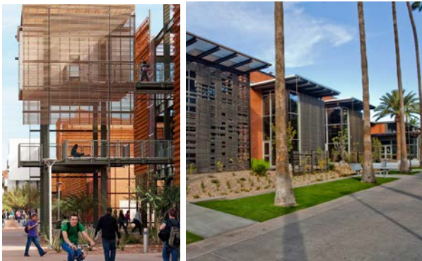
Articulation of buildings façades enriching the campus environment and providing human-scale comfort at eye-level.
