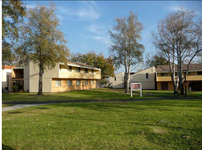
SERRANO VILLAGE Setting and adjacency of buildings within the cluster.
