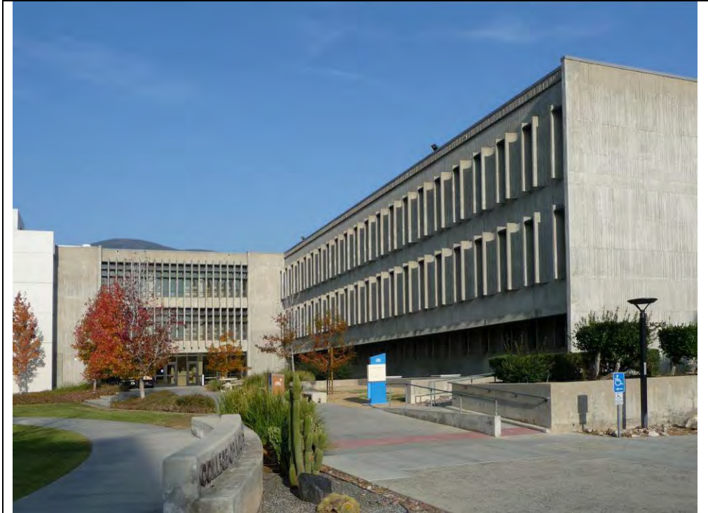
Biological Sciences building, 1967, main facades view north.
