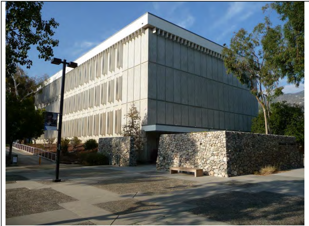
Physical Sciences building, 1967, as approached from Library, view northwest.
