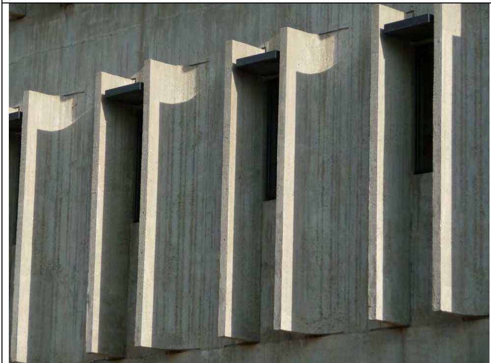
Biological Sciences, detail of concrete finish and "fins" at windows, west façade.
