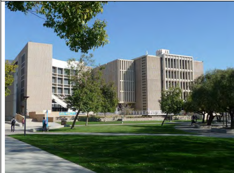
JOHN M. PFAU LIBRARY General view northeast from quad with addition at left.
