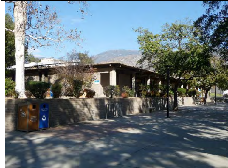
SIERRA HALL View north from parking lot entrance; building elevated on retaining wall.
