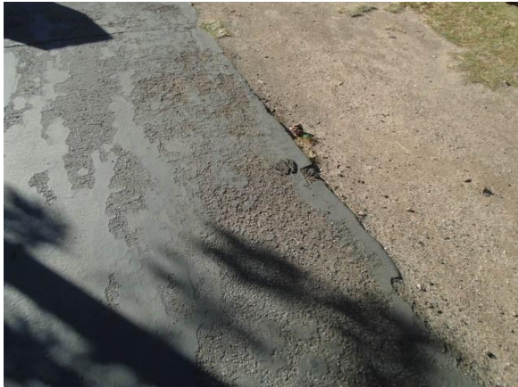
MCADA008a Main Campus Site Deteriorating asphalt pedestrian pathway Serrano Village
