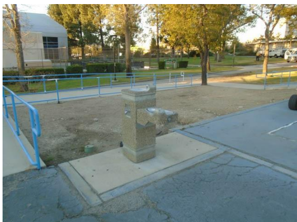
216007a Temporary Kinesiology Annex Accessible dual-level drinking fountain South exterior
