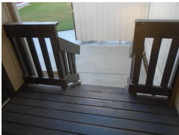
115-A006a Univ Ctr for Dev Disabilities Steps with noncompliant handrails Breezeway entrance area
