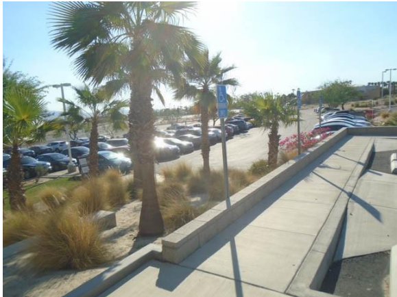
PDADA012a Palm Desert Campus Site Accessible parking, curb ramp and compliant signage South of Indian Wells Theater
