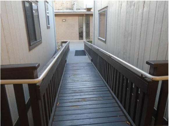
115-A003a Univ Ctr for Dev Disabilities Entrance ramp with accessible handrails on both sides Breezeway entrance area
