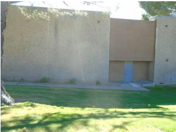
MCADA017a Main Campus Site Ramped sidewalk without the required handrails North of the theater building
