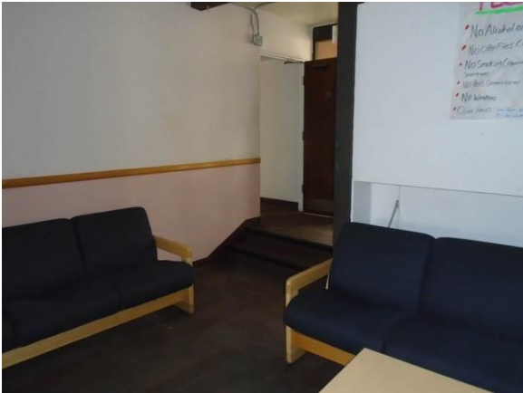
017014a Badger Residence Hall Main lobby steps without required handrails Room 100
