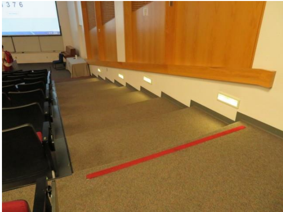
032043a Visual Arts Center Nongraspable wall railing in auditorium Auditorium
