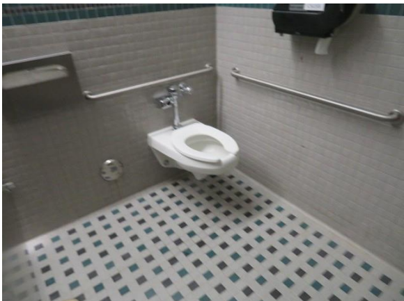
032068a Visual Arts Center Accessible water closet with grab bars Ceramics building, men's restroom
