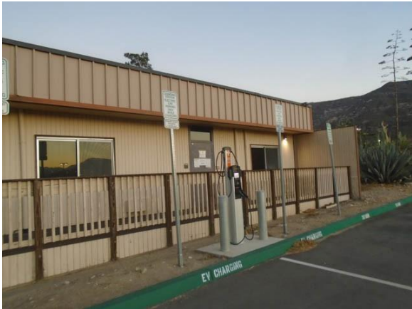
301-2001a Temporary Classrooms Building exterior and site conditions East exterior
