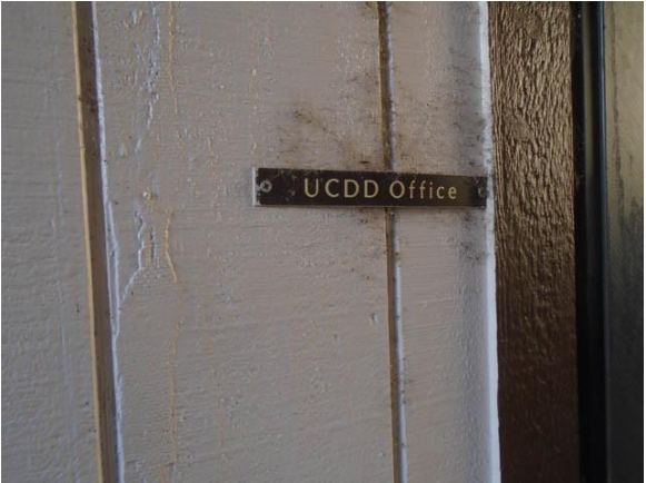
115-A001a Univ Ctr for Dev Disabilities Nonaccessible signage, typical Breezeway entrance area
