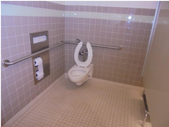
020040a Performing Arts Accessible water closet with grab bars Restroom MR137A
