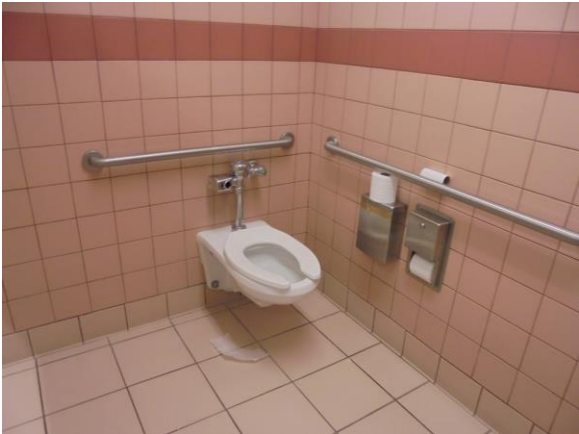
001010a Administration ADA water closet stall Restroom WR124
