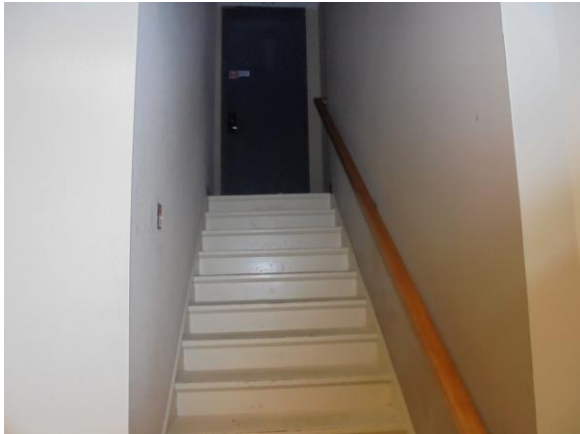
020026a Performing Arts Steps with single handrail First floor
