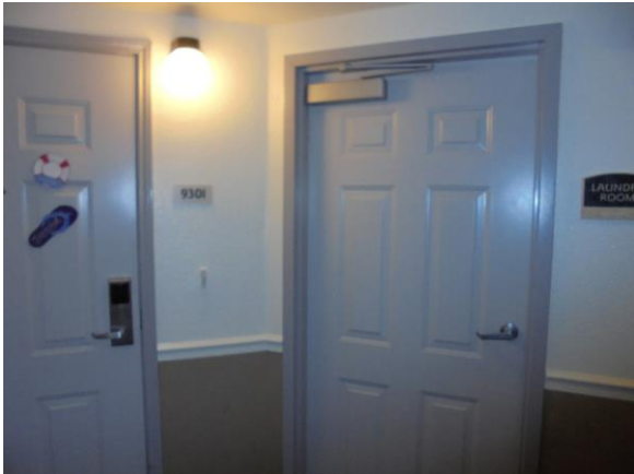
075005a University Village Housing Corridor doors with lever hardware and Braille signage Building 9, third floor
