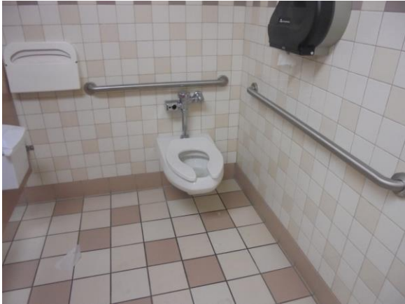
007010a Biological Sciences Accessible water closet with grab bars Restroom WR301
