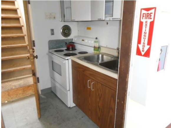
017023a Badger Residence Hall Kitchen with nonaccessible casework and sink Room 224
