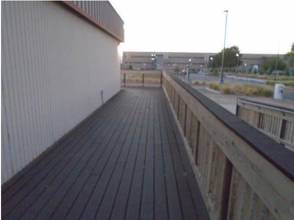
301-2002a Temporary Classrooms Porch area outside TC-302 South exterior
