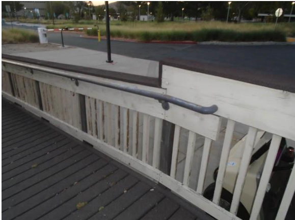
301-2005a Temporary Classrooms Accessible ramp to the porch area South exterior
