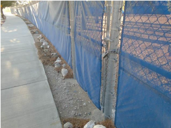
MCADA013a Main Campus Site No accessible entrance into the Leadership Challenge Center Leadership Challenge Center
