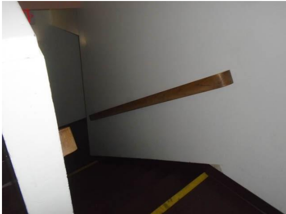
017019a Badger Residence Hall Stair with noncompliant handrail Stairwell
