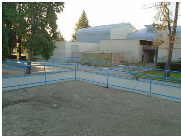
216004a Temporary Kinesiology Annex Ramp to the building main entrance South exterior
