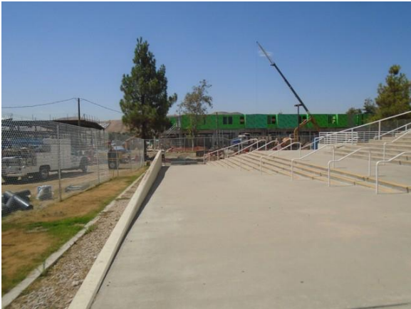
MCADA019a Main Campus Site Ramped walkway without required handrails East side of Jack H. Brown Hall
