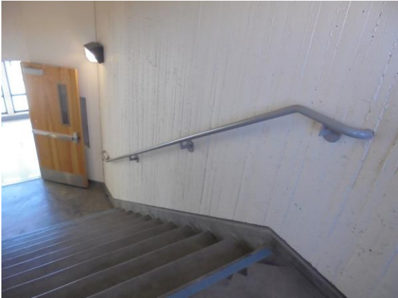
007008a Biological Sciences Compliant stair handrail design Third floor
