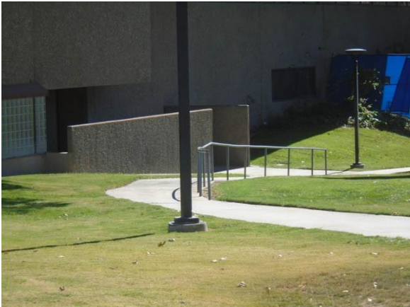
MCADA001a Main Campus Site Ramped sidewalk without required railing West of the theater building
