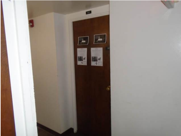
017021a Badger Residence Hall Typical sleeping room door with nonaccessible signage and hardware Second floor
