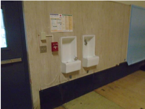
010054a Physical Education Nonaccessible drinking fountain in the gym Room 100
