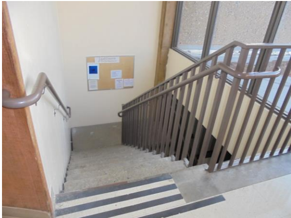
020024a Performing Arts Compliant stair handrail design Second floor
