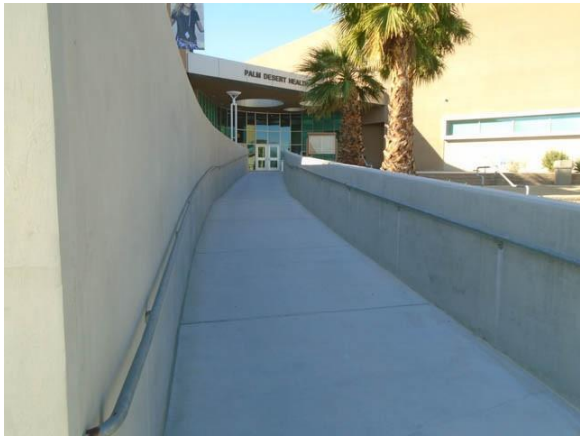
PDADA008a Palm Desert Campus Site Compliant accessible ramp East of Health Sciences
