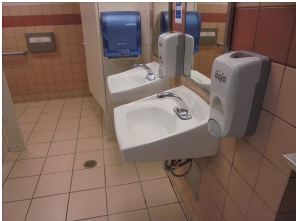
001009a Administration ADA lavatories Restroom WR124
