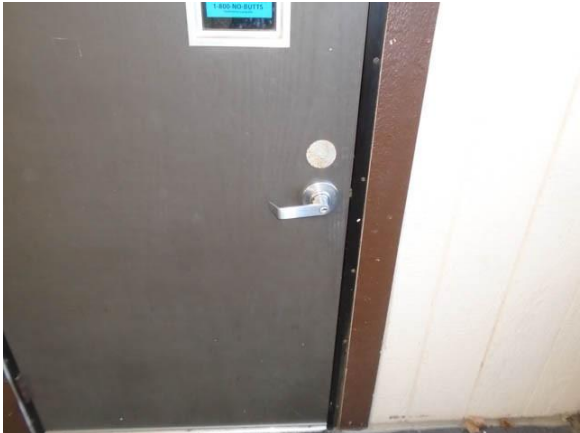
115-A002a Univ Ctr for Dev Disabilities Accessible door hardware Breezeway entrance area
