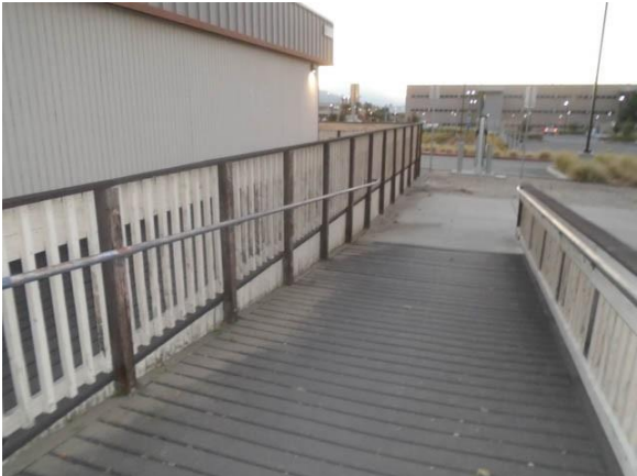
301-2004a Temporary Classrooms Accessible ramp to the porch area South exterior
