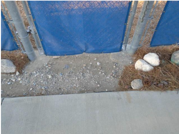
MCADA014a Main Campus Site No accessible entrance into the Leadership Challenge Center Leadership Challenge Center
