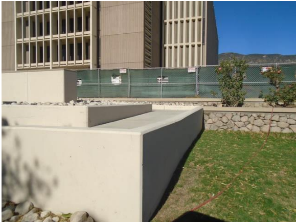
MCADA002a Main Campus Site Ramp not required to have a handrail South of Pfau Library
