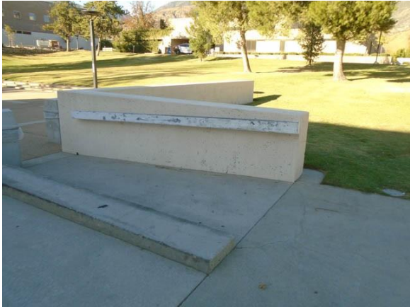
MCADA004a Main Campus Site Noncompliant handrail at a ramp West of the Commons
