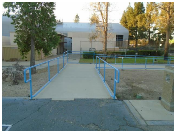
216006a Temporary Kinesiology Annex Top of the ramp with accessible handrails South exterior
