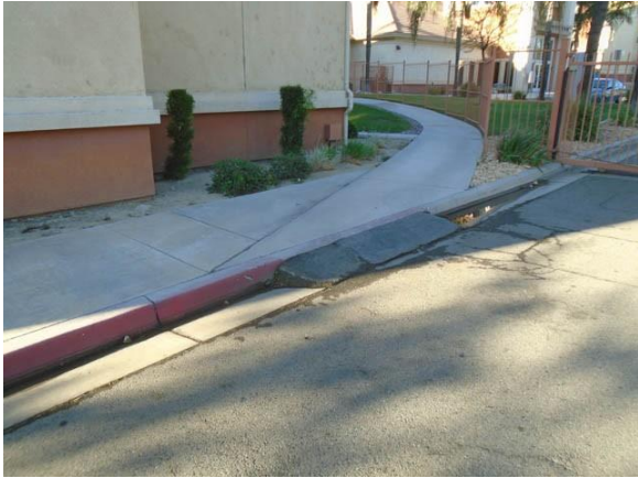
MCADA006a Main Campus Site Improper ramp at curb East side of University Village
