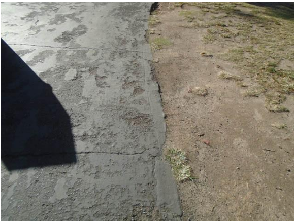
MCADA009a Main Campus Site Deteriorating asphalt pedestrian pathway Serrano Village
