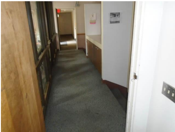
014009a Mojave Residence Hall Entry steps lacking handrails Room 100
