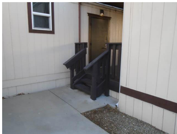
115-A007a Univ Ctr for Dev Disabilities Steps with noncompliant handrails Breezeway entrance area
