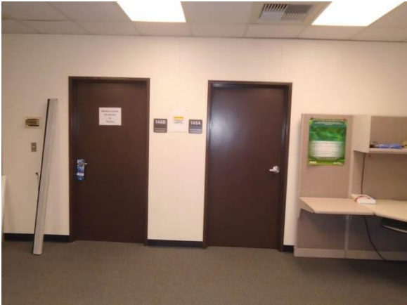
301-2012a Temporary Classrooms Interior doors with accessible signage and hardware Room 146
