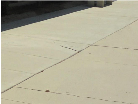
MCADA020a Main Campus Site Trip hazard Between Administration and Chaparral
