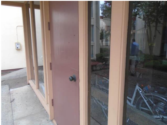
014007a Mojave Residence Hall Door with nonaccessible hardware at the entrance vestibule North elevation
