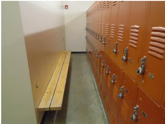
010039a Physical Education Lockers and bench without accessible features or clearances Locker room 148
