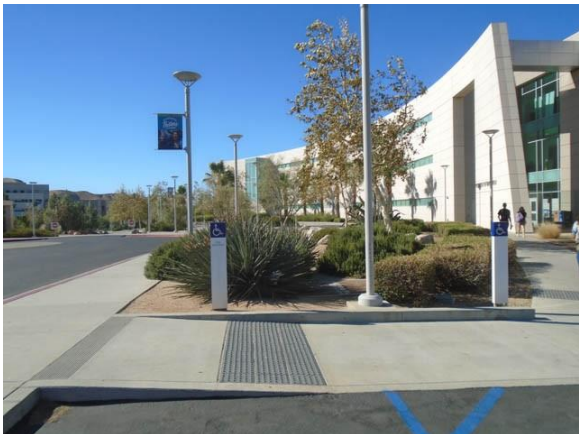
MCADA018a Main Campus Site Signs below required height Education Building
