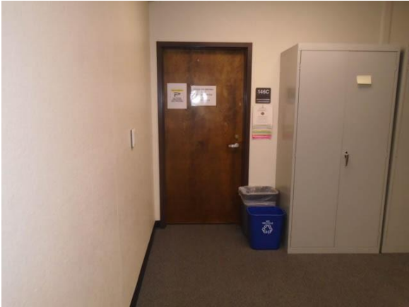
301-2008a Temporary Classrooms Typical interior Room 146
