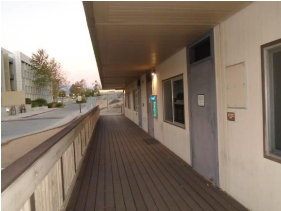
301-2006a Temporary Classrooms Porch area at Module TO-301 South exterior
