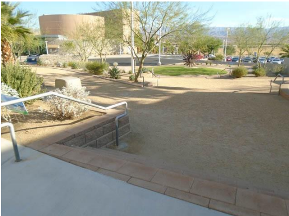
PDADA009a Palm Desert Campus Site Stairs with compliant handrails East of Health Sciences
