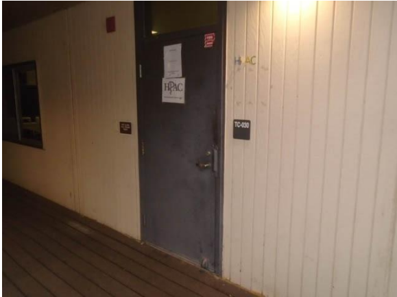
301-2003a Temporary Classrooms Typical entrance door, Module TC-302 South exterior
