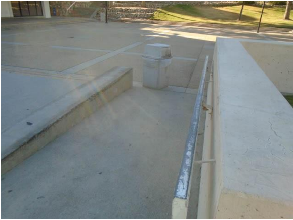
MCADA005a Main Campus Site Ramped sidewalk without required railing West of the Commons
