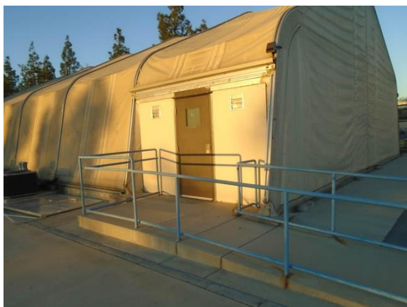
216001a Temporary Kinesiology Annex Accessible entrance/exit ramp at the building rear door East exterior
