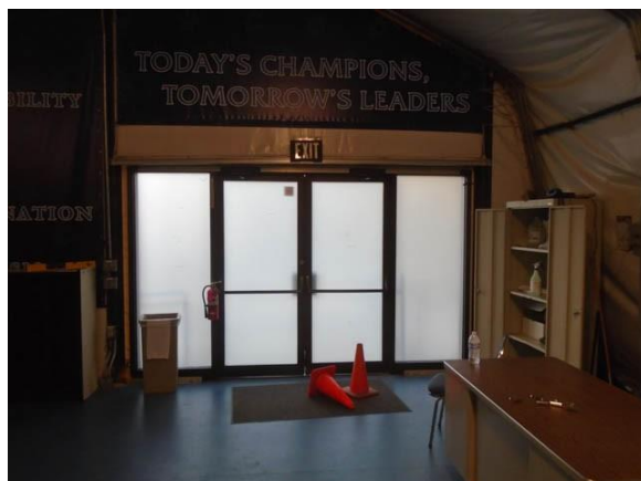
216008a Temporary Kinesiology Annex Main entrance door and hardware Interior
