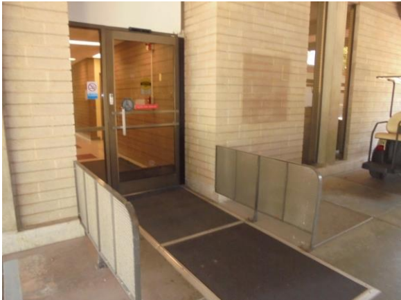
001031a Administration Power assisted entrance South elevation
