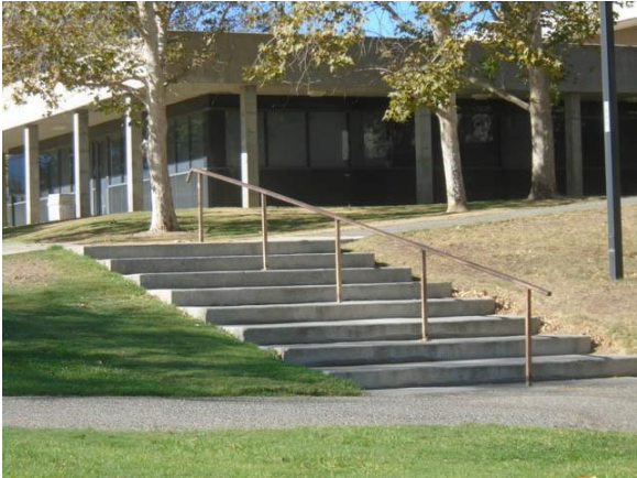
MCADA003a Main Campus Site Stair without required handrail on both sides Southeast of Pfau Library
