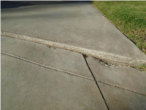
MCADA007a Main Campus Site Noncompliant level change, trip hazard South of Yasuda Center
