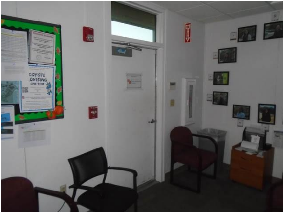
301-2013a Temporary Classrooms Entrance door with accessible hardware Room 031
