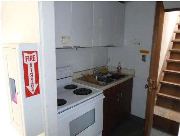
014013a Mojave Residence Hall Common area kitchen with noncompliant casework Room 224
