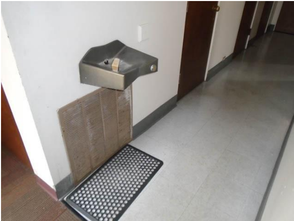
017033a Badger Residence Hall Single-level drinking fountain First floor
