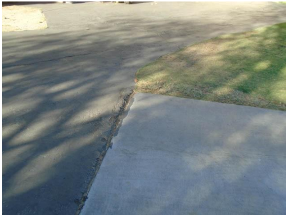
MCADA010a Main Campus Site Deteriorating asphalt pedestrian pathway Serrano Village
