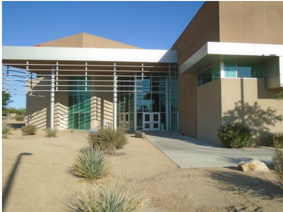
PDADA006a Palm Desert Campus Site Accessible route from the accessible parking area Health Sciences
