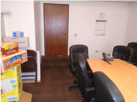
017013a Badger Residence Hall Meeting room with noncompliant door hardware and steps without required rails Room 119
