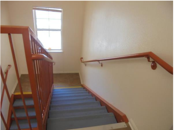
075007a University Village Housing Compliant stair handrail design Building 9, third floor
