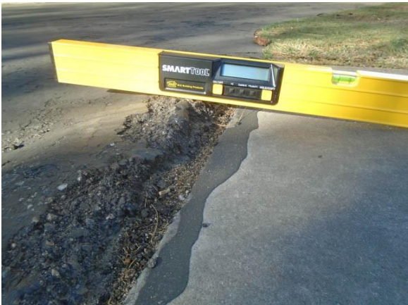
MCADA011a Main Campus Site Deteriorating asphalt pedestrian pathway Serrano Village
