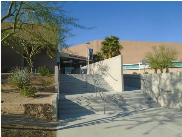
PDADA007a Palm Desert Campus Site Stairs with compliant handrails East of Health Sciences
