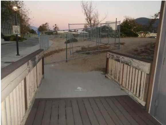
301-2007a Temporary Classrooms Grade-level entrance to the porch at TO-301 South exterior
